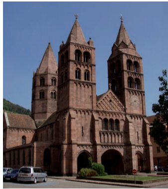
Saint-Léger church, built under the Murbach abbot princes at the end of the 12 th century
