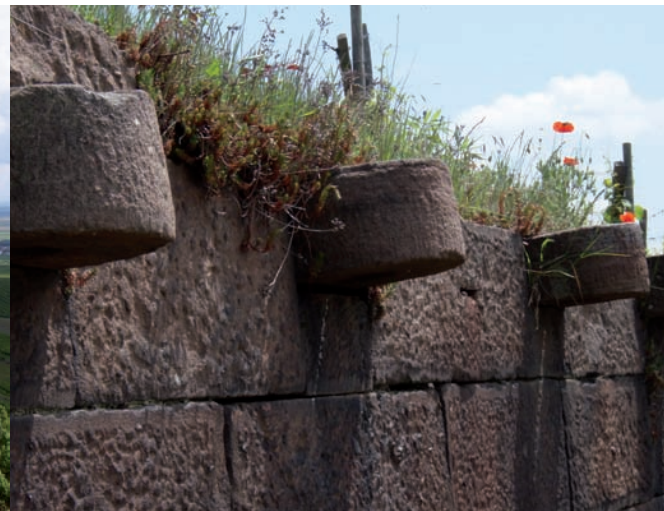
Half-moon stones, crossed with a wooden stake, allowing the planting of one last vine right above the wall.
